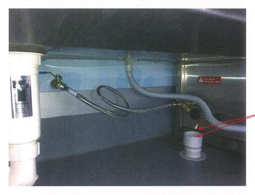
Tundish with air gap between the copper pipe and tundish highlighted.
