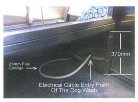
The above picture shows the main electrical cable entry point into the dog wash. Once you have run the cable and conduit to this point, leave another 900mm for the termination inside the cabinet.
