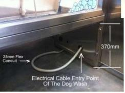
Shown on the left is a photo of the main electrical cable entry point to the dog wash. Once you have run the cable and conduit to this point, THEN leave another 900mm for the termination inside the dog wash.
