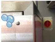
Shown on the right is the main electrical cable inside the dog wash. It enters through the gland at the bottom of the dogwash close to the ground. Run the power cable in 25mm flexible conduit as there is a socket already installed into the bottom of the main circuit breaker box shown. Leave 1m in length after you have reached the bottom gland.
