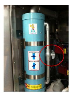
NOTE: Set for summer operation when the weather is consistently warm and above 30deg C (86deg F)
