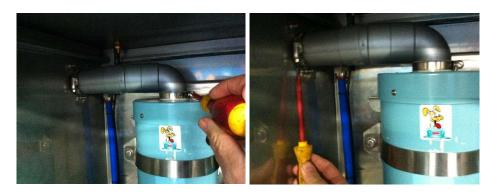
Please note heated dryers only have the one clamp but have a screw that needs to be tightened.
