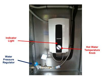
The DHCE 8/60 fully electronic instantaneous water heater heats the water while it is flowing through the unit. The indicator light will show when the heater is operation.
