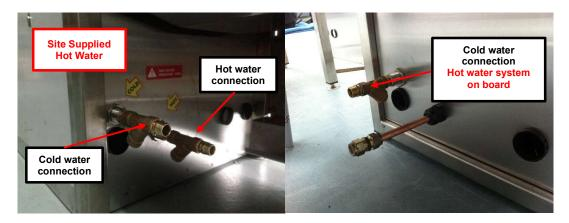
Once connected the regulator can be adjusted to ensure the K9000 has water pressure of between 20 & 30 psi when the pressure gun is in use and between 40 & 50 psi when pressure gun is not being utilised.
