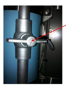
Set the Dryer bypass tap to the position as shown for **SUMMER** operation.
