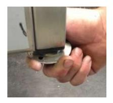
Now place the right and tub as near as possible to the left-hand tub, place a level along the back of the Dog Wash and adjust the feet according to get the Dog Wash Level. This will help assemble the two pieces.
