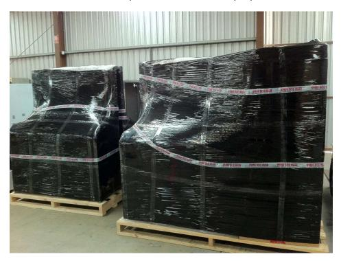
Position the Dog Wash while on the pallets near their final location. The larger section of the Dog Wash goes to the left-hand side, with the highest point being the back of the Dog Wash. Take caution removing the plastic and bubble wrap avoid using a knife as it may scratch the stainless steel or decals. With a screw gun remove the screws from the feet and the tie down straps.
