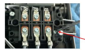
Activate the safety pressure limiter for flow pressure by firmly pressing in the reset button (the appliance is delivered with the safety pressure limiter disabled).
