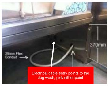
The picture above right shows the main electrical cable entry point into the dog wash. Once you have run the cable and conduit to this point, leave another 1500mm for the termination inside the cabinet.
