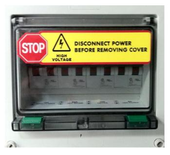
Each of the safety circuit breakers are "doubles' and this is reflected in the labelling of the Breaker Box.
