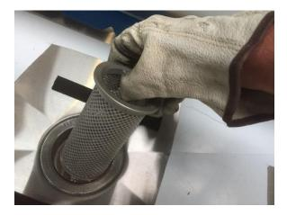
While the filter is removed, place the wash gun in the drain, set the wash gun to "JET", Key Pad selection to RINSE (option 2) and flush the drain. Run the water gun for 20 seconds, if there are issues with the water draining away you may need to contact your plumber. Replace the cylindrical filter and put the stainless-steel filter back into position.
