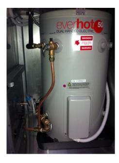
2.2.2.3 Shown picture below shows the water entry point for a K9000 2.0 with a hot water storage service.
